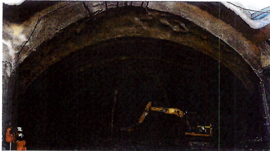
Example of tunnel with top bench in three phases
